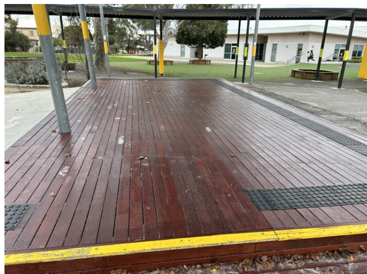
Repainted Prep Deck
